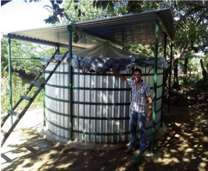
Fig. 5 Impluvium tank with roof and gutters. Source IDE (2017)
