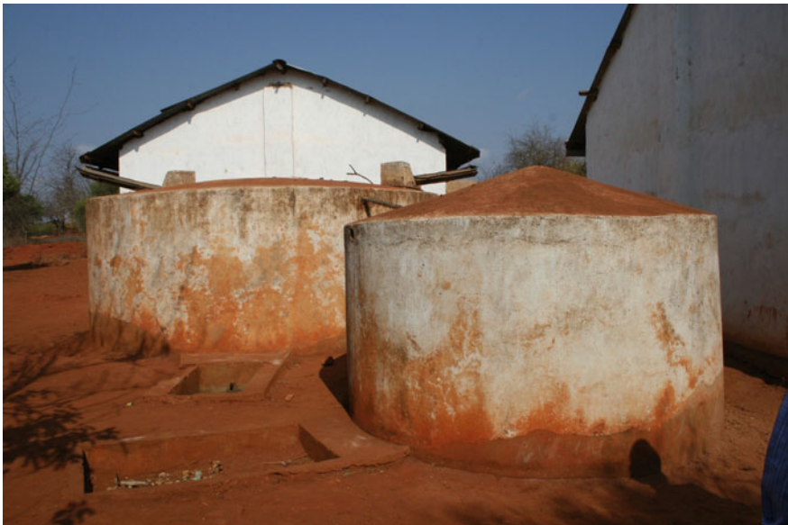
Fig. 4 Roof catchment system with ferro-cement tanks. Photograph Josep de Trinchera Gomez
